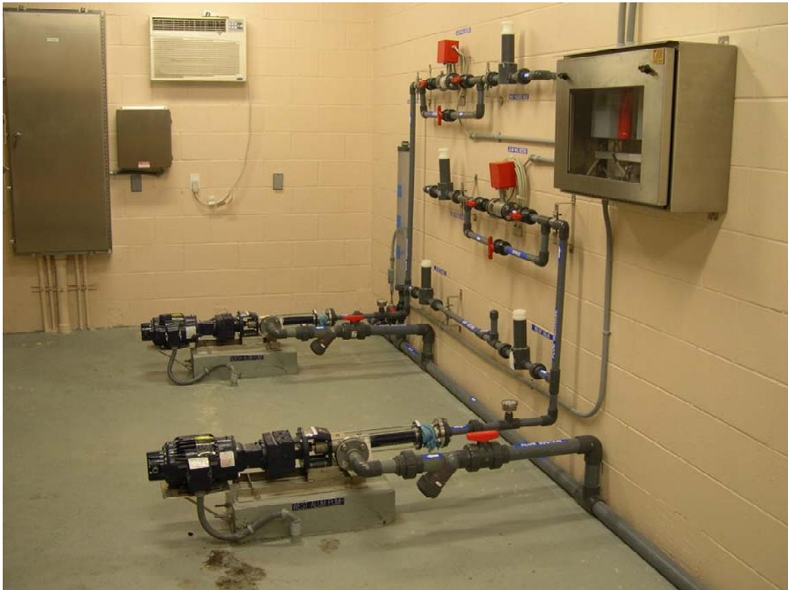
Figure 2-5. Overview of Alum System Pumping and Piping.
