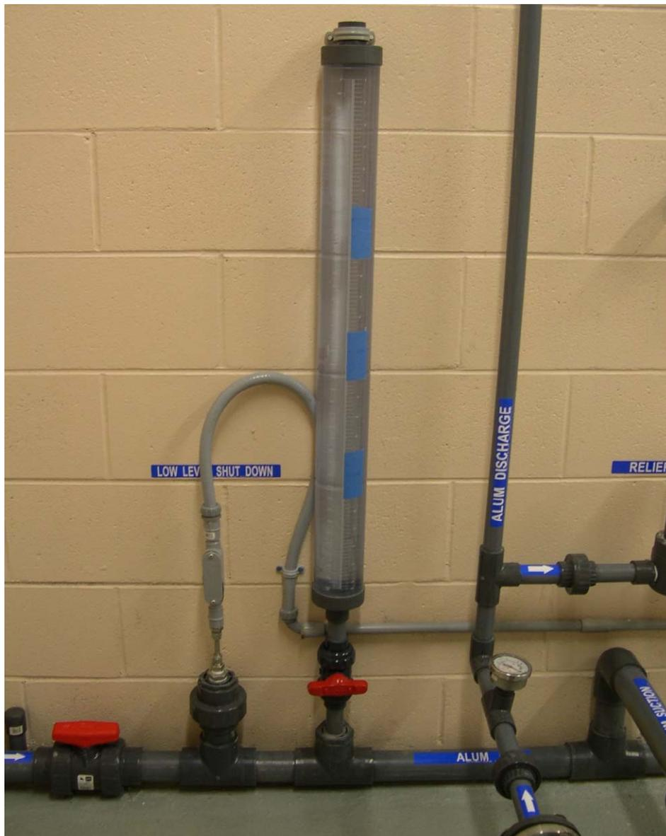
Figure 2-6. Alum Pump Calibration Chamber.
