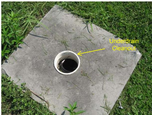
Underdrain Clean-out Structure
