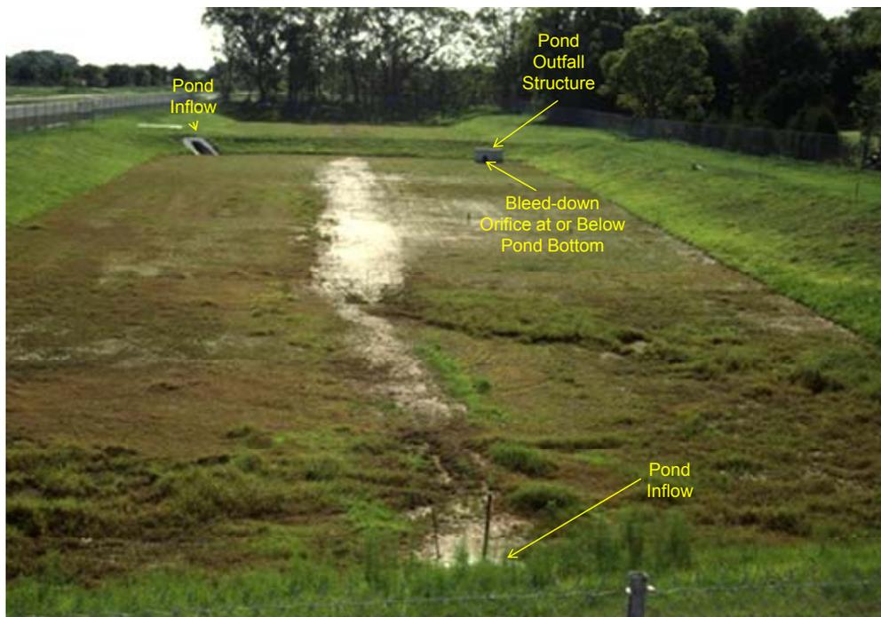
Figure 2-2. Photograph of a Typical Dry Detention Pond System.
