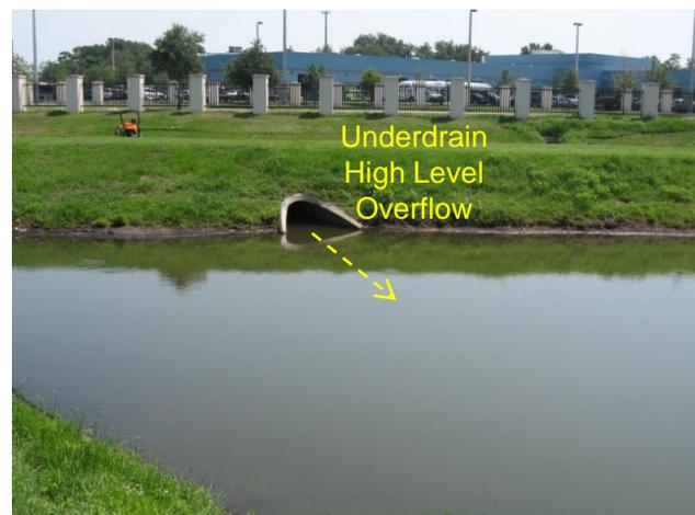
Site 5 – Underdrain High Level Overflow to Wet Pond
