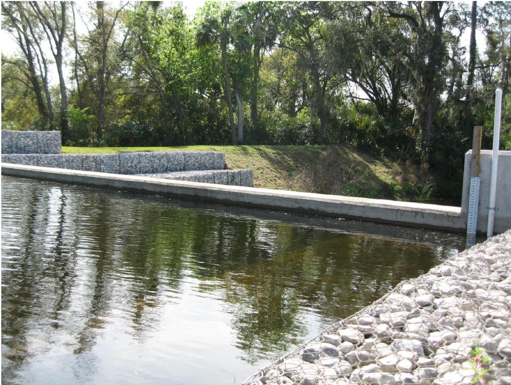
Figure 1-6. Diversion Weir/Overflow Spillway.
