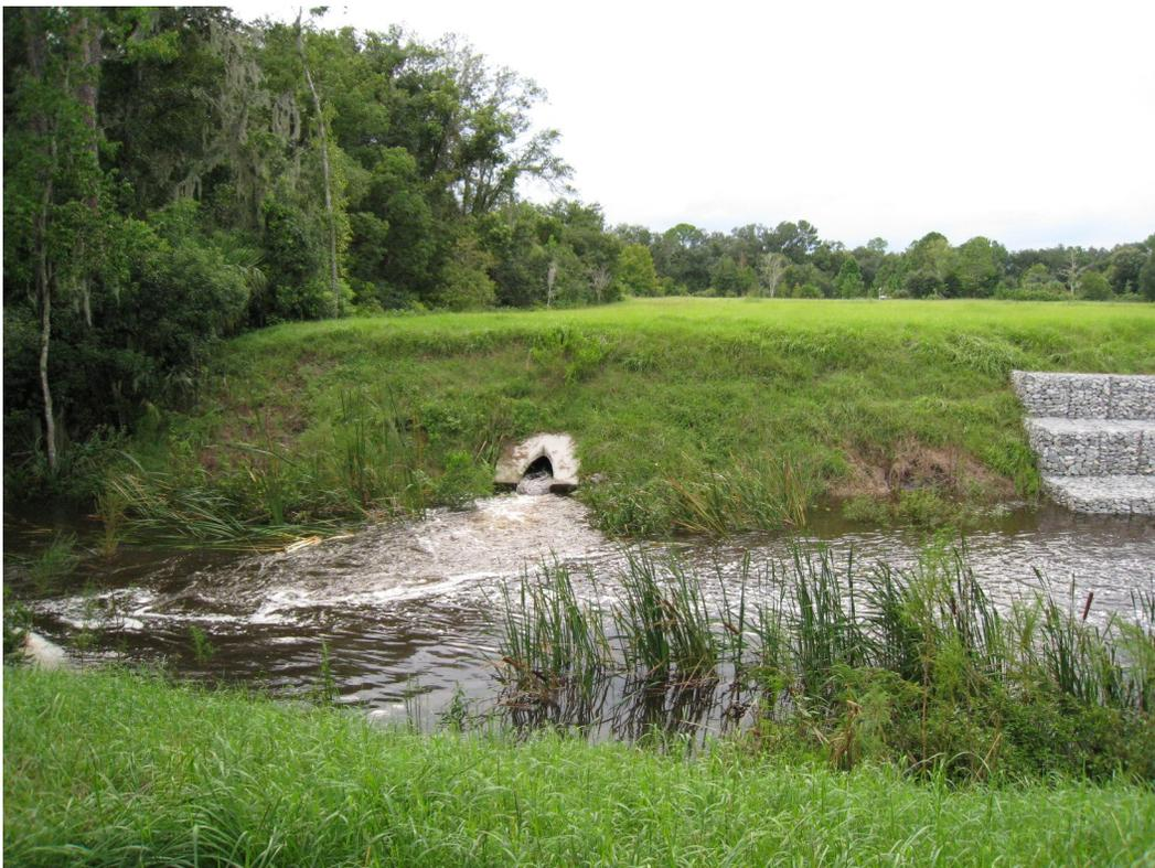
Figure 1-7. Pond Outfall through 24-inch RCP.
