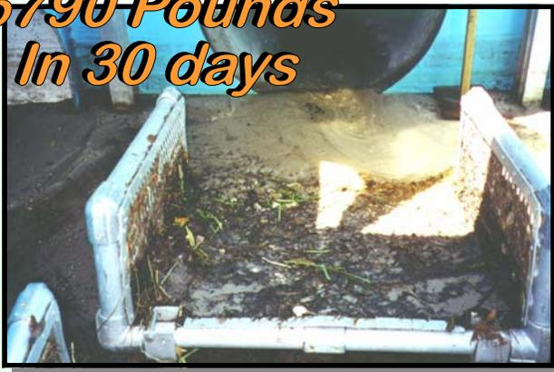
To the left is a view of 5790 pounds of sediment collected in a *Nutrient Separating Baffle Box* just 30 days after installation.
