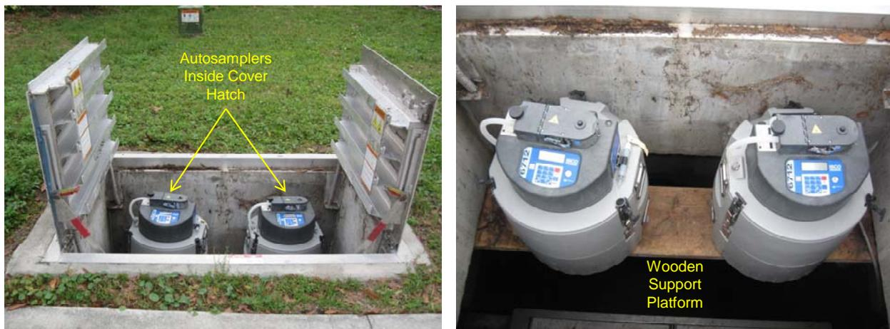
Figure 3-3. Overview of Sampling Equipment Installed at the Gee Creek Site.
