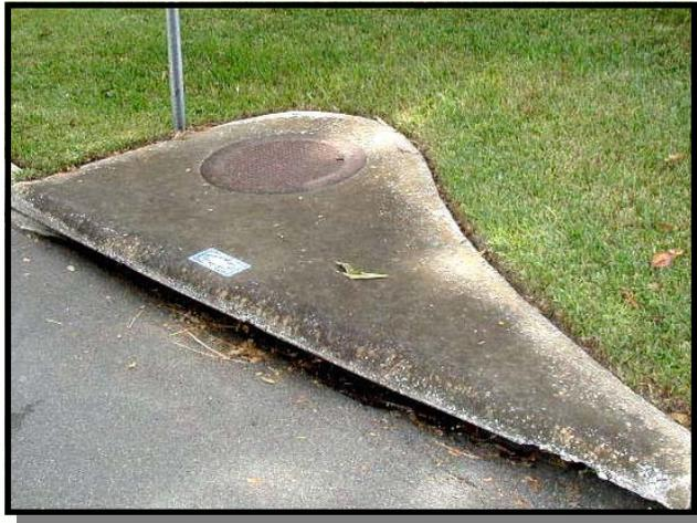
**Above:** View of the curb inlet showing that the only access is through a manhole.
