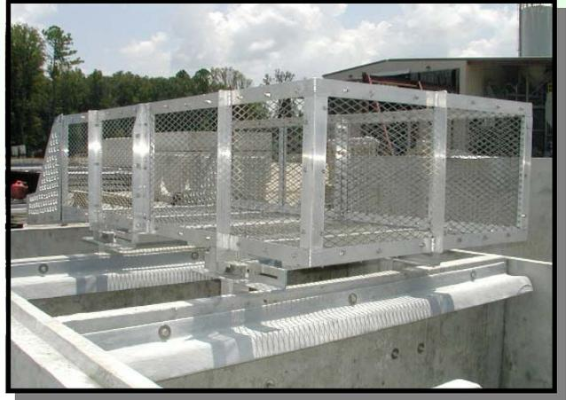
**Turbulence deflectors are attached to the tops of the baffles with stainless steel bolts. Several bolts per deflector are required.**
