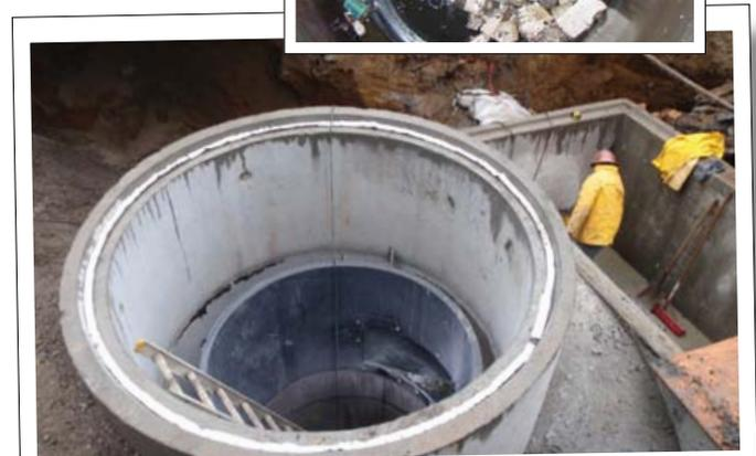
*CDS unit installed to remove trash before entering Lake Meritt in Oakland, CA*
