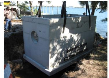
EcoVault® treats the continuous flow while debris screens span the entire box, creating extensive storage volume.
