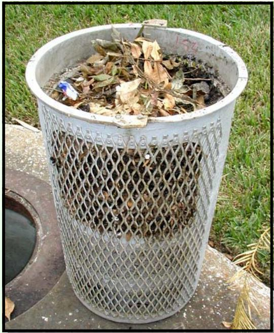
**Left:** The **Curb Inlet Basket** has been removed and can be easily emptied by hand without the need of a vacuum truck.
